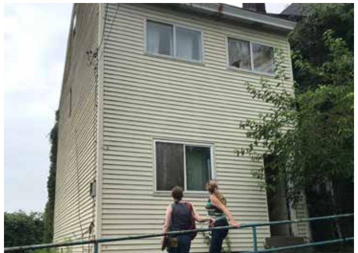
The action plan prioritizes properties already under FCC/PHCC site control, such as 9 Lanark Street, which has a full renovation plan underway. Photo by SfSP.
