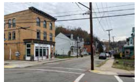
Perryville Avenue mixed-use buildings; Wilson Street view
